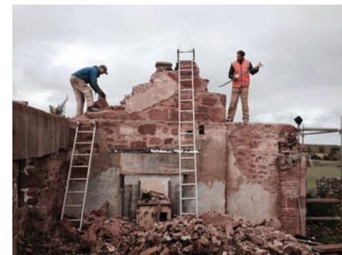
had fallen in, the internal walls had collapsed, the windows were either missing or beyond repair and the external stone walls and chimneys needed a bit of repair work."
