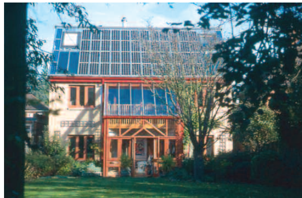
4KW (approximately 30m 2 ) PV array yielding 3,000 KWh/yr at the Oxford Eco-House. Photo courtesy of Sue Roaf
