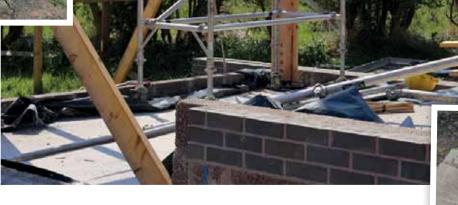
measurements, to ensure that the setting out, and levels, of the bases were correct. This was the second time this had been done, as Luke was on site to measure the dimensions before the frame was started in the workshop. As Luke says, 'Measure twice, cut once.'
